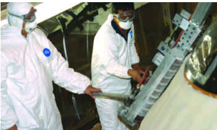
Lockheed Martin's Ken Phillips (left) and Toan Nguyen use the new portable "pencil sharpener" tool to trim and machine the foam spray repair on ET-124's forward ogive. The tool, designed and built in 10 days specifically for the repair at Kennedy Space Center, performed flawlessly.
