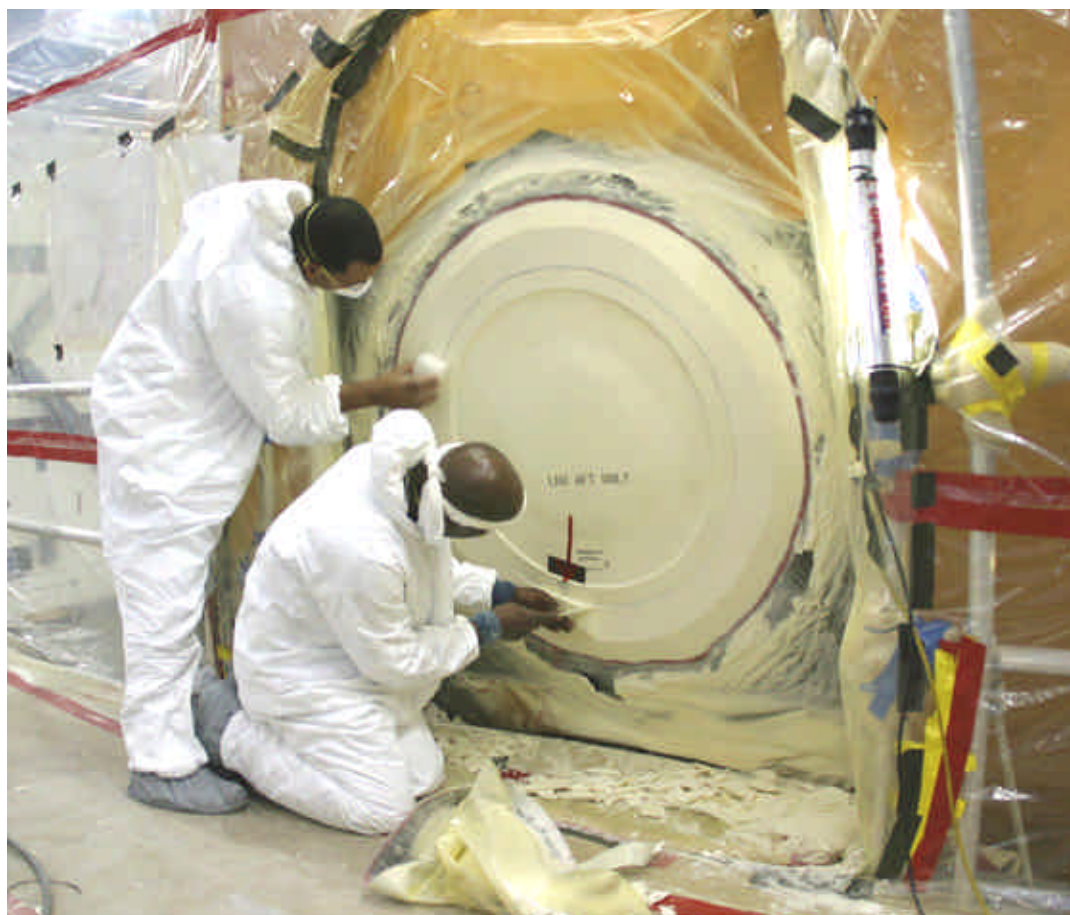
Technicians Troy Smith (left) and Joe Johnson trim foam on the manhole cover of ET-118 at Kennedy Space Center.
